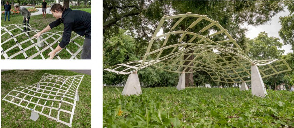
圖32：Design and fabrication of multi-patch elastic geodesic grid structures[55]
