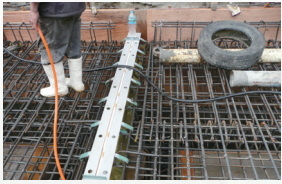
27 橋梁伸縮縫安裝
