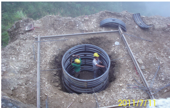
墩柱區井筒式基樁(人工手掘式)鑽掘
