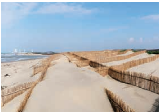
▲苑裡苑港段堆砂籬
