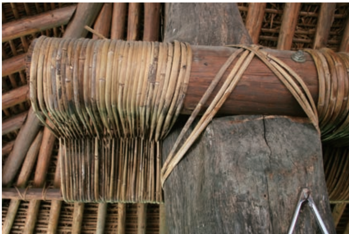
家屋的樑柱採用黃藤皮固定 iving houses are fixed by barks of yellow rattan palm.
