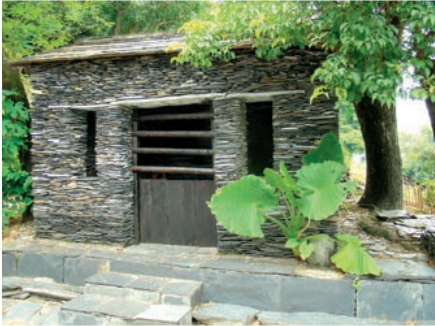
牲畜房 The livestock house.
