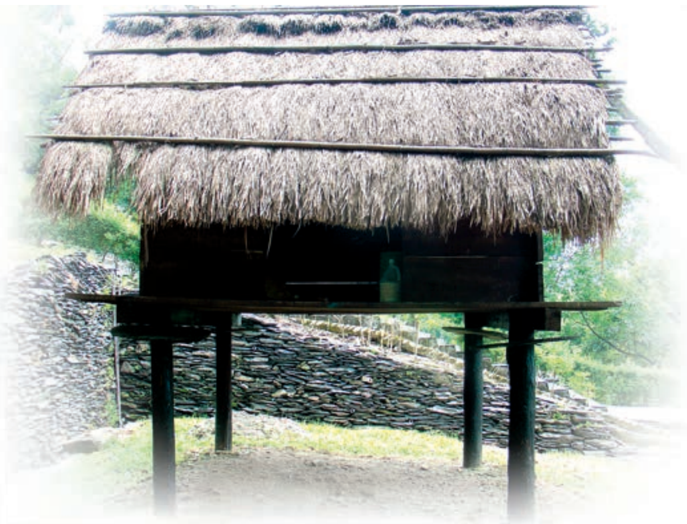
穀倉角柱與高床平版間設有防鼠板也可為建材短料繩 The rat preventing boards are installed on prisms just below the floor.
