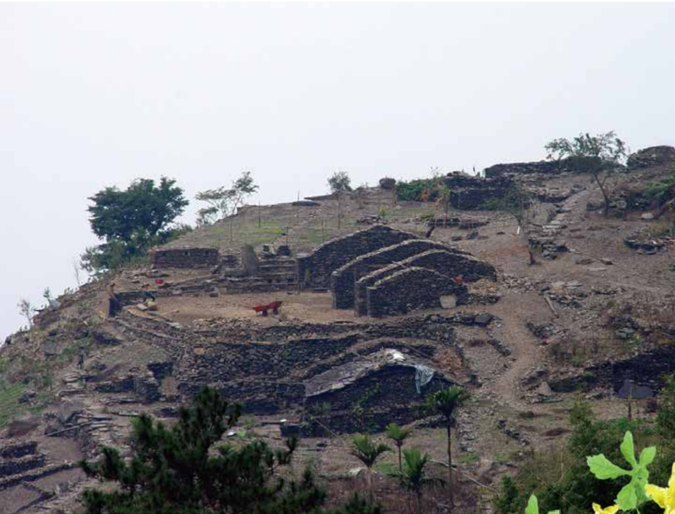
重建中的石板屋 The shale stone houses in rebuilding.
