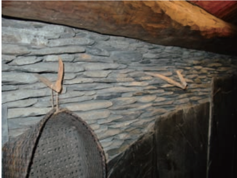
石板屋之內壁 Wall of shale stone house.
