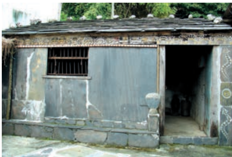
石板屋正面圖 Front view of shale stone house.
