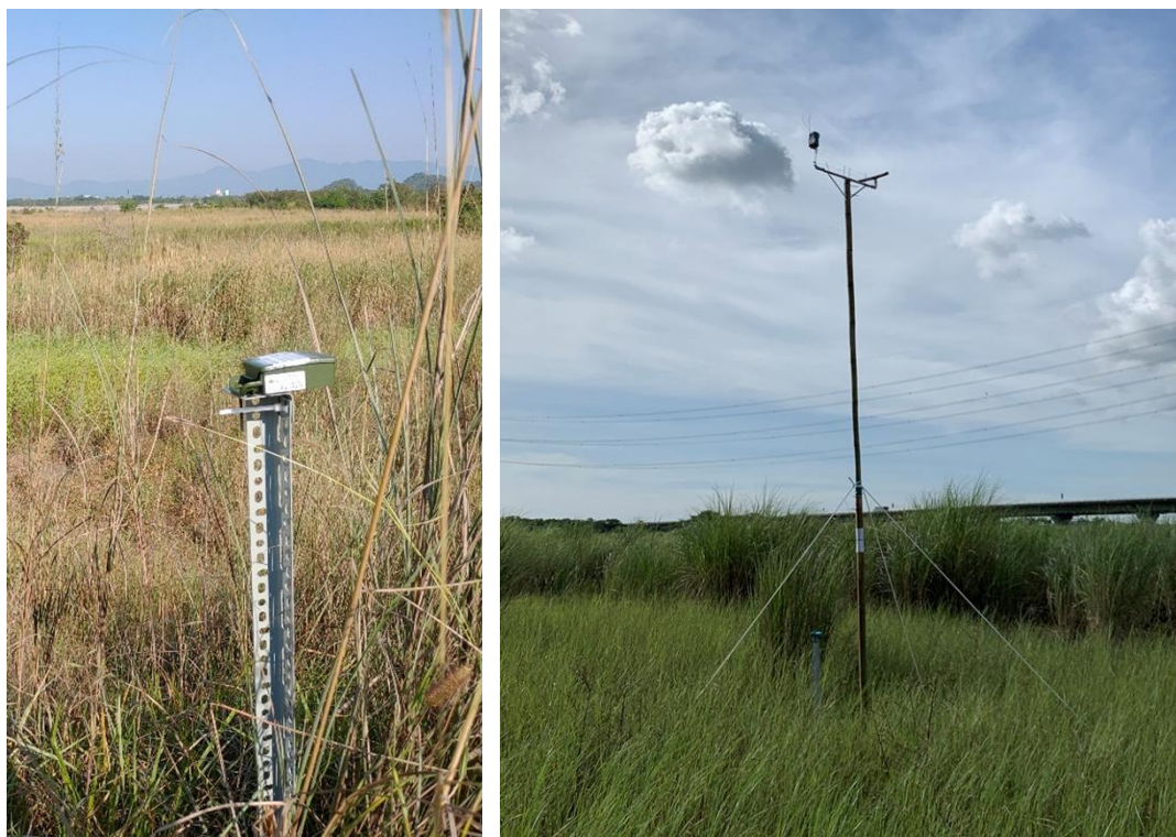
Figure3. Example of recorder installation in the field.
